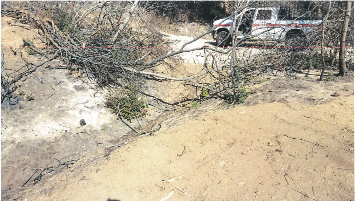
Photo taken 11-6-2020 by R. Sampson. Photo point RS-5 looking east upslope. Shows Class III drainage with new rocky crossing but lower right is uncontrolled bare filled created during operations. Drainage across this fill (see next photo) is all directed down its length into the watercourse channel without breaks or filter.
