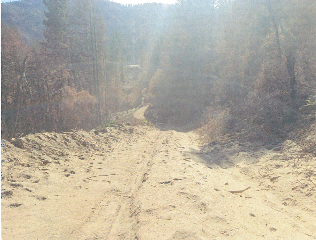
Photo taken 11-4-2020 by S. Bullock Photo Point SB-2. Shows lack of road watering and waterbars on seasonal road. Note, this road segment is on Big Basin Water Co. Lands in the Boulder Creek watershed above numerous water intakes and Coho and Steelhead habitat.
